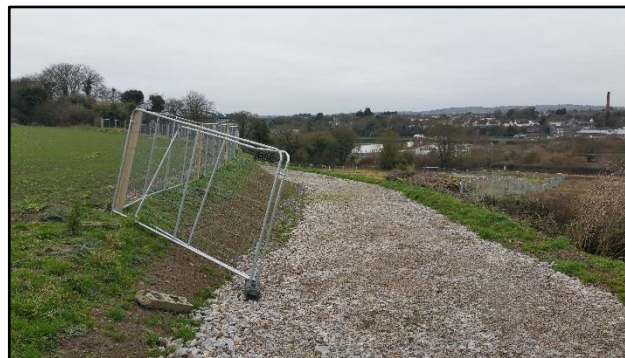
Figure 10– Temporary Construction Access leading to site of P.A. Ref. No. 17/387
