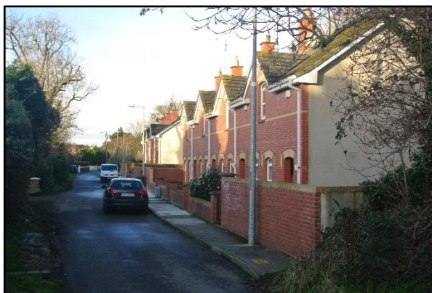
Figure 15 - View south along Railway Terrace
